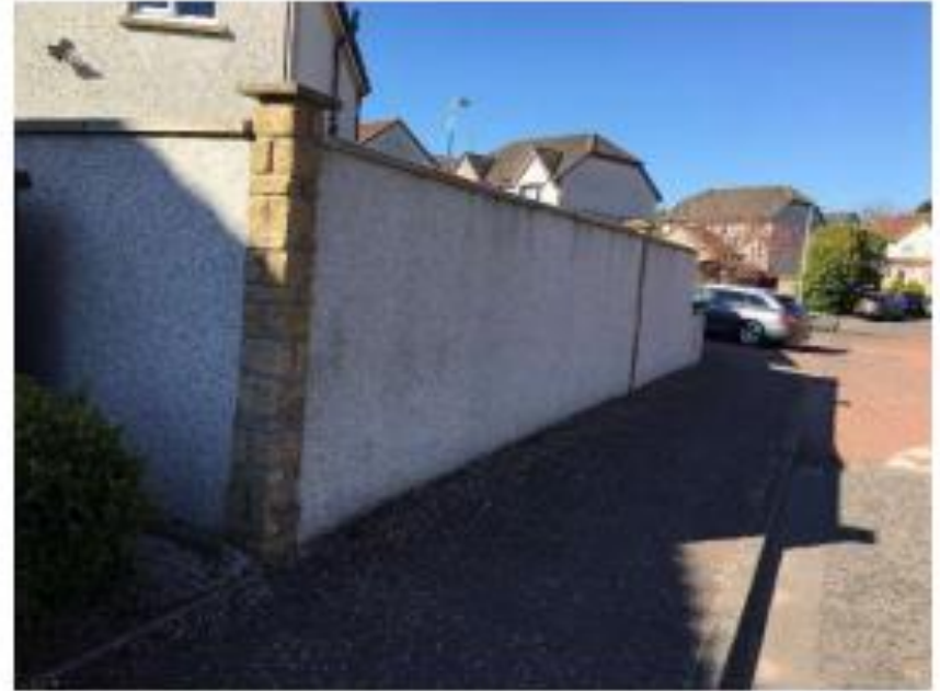
Photograph No. 14 Wall at 48 Seaview Place
